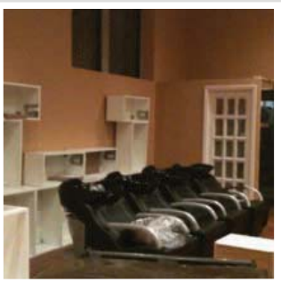
Renovation in Progress
